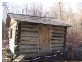
Richard Muny Chemsultants Blacksmith Shop
